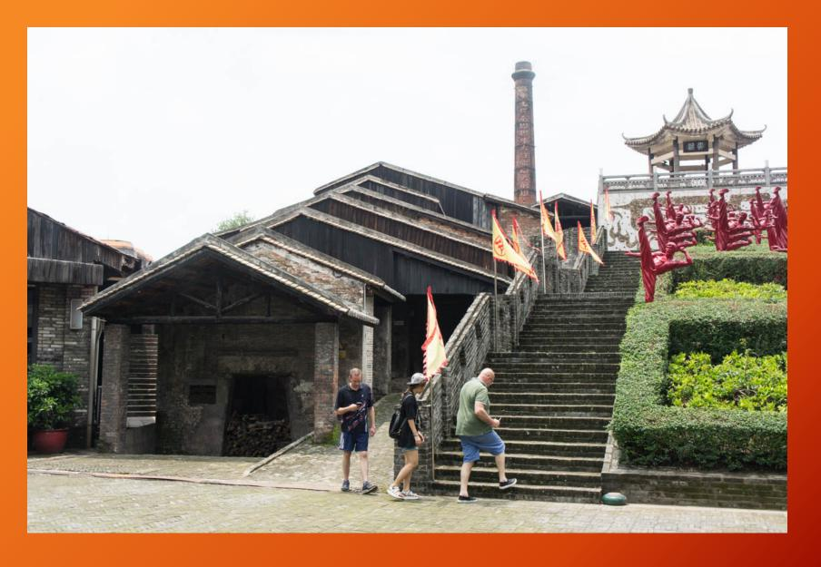
This side view of the High Kiln shows the climbing nature of the dragon kiln which is covered by the stepped roofing sections to protect the kiln roof from the elements.
