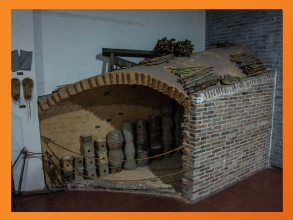
Cross-section of a dragon kiln firing tunnel.
